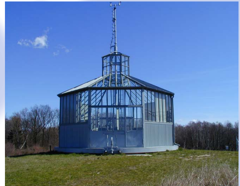
The winch house at Lindenberg Observatory: Technical monument for the operational launch of meteorol. kites in the last century
